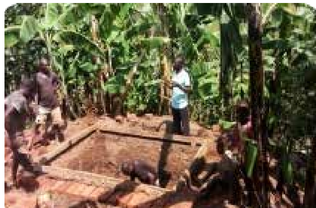
Figure 1: A Community Mobiliser training community members on underground water tank construction, Kabale cell in Kabale District.
